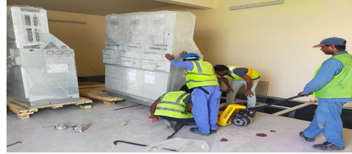
11KV MV SWITCHGEAR PANEL INSTALLATION AT PROJECT: COSMOPLAST FACILITIES AT KIZAD
