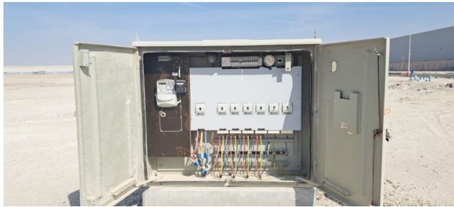
STREET LIGHTING CONTROL PANEL, AL MARKAZ INDUSTRIAL PARK, DHFRAH
