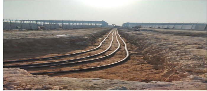
11KV 3x400MM2 CABLE LAYING WORKS AT PROJECT: COSMOPLAST FACILITIES AT KIZAD
