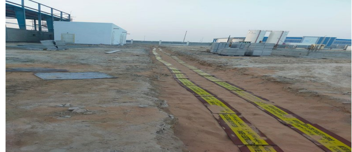
11KV CABLE PROTECTION TILES INSTALLATION AT COSMOPLAST PROJECT, KIZAD
